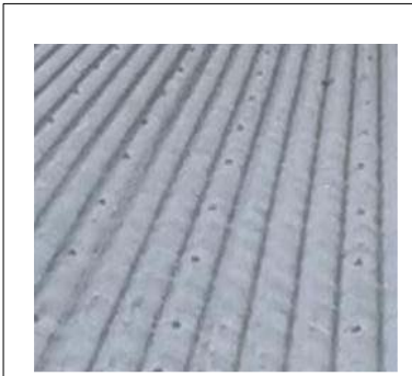
EXISTING ROOF SHEETING
